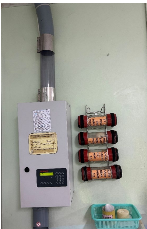
Figure 3: Pneumatic tube system for sending mother and infant delivery samples
