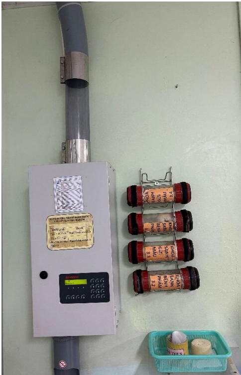
Figure 4: Pneumatic tube system for sending mother and infant delivery samples
